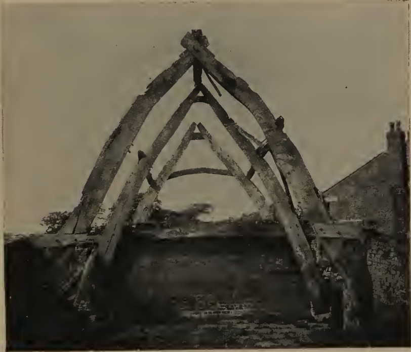
The frame of a wattle and daub house of a labourer
